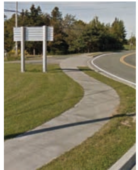
FIGURE 5.15 Apron Driveway Treatment for Separated Bike Lane
