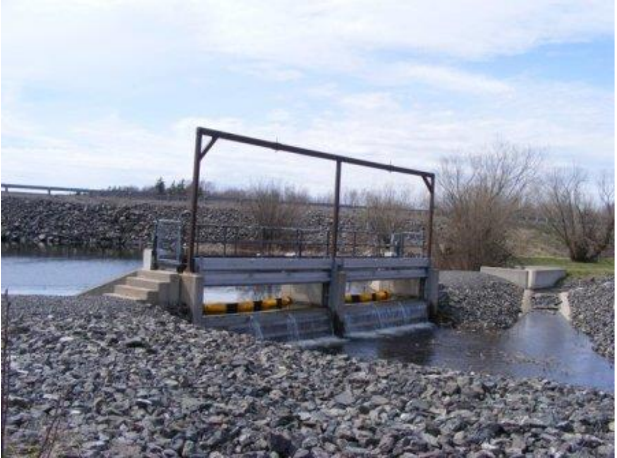
Figure 3. Stop logs and eel weir adjacent to Pottle Lake pump house
